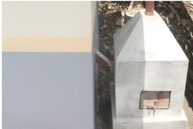
Female toilets in secondary schools were equipped with incinerators to dispose sanitary pads.
