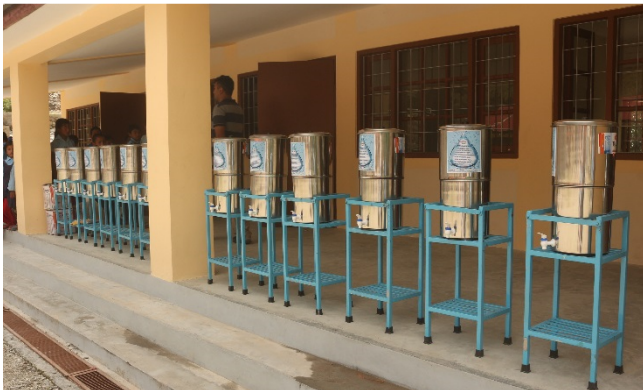
Drinking water tanks with integrated colloidal silver filters were provided in schools where needed.
